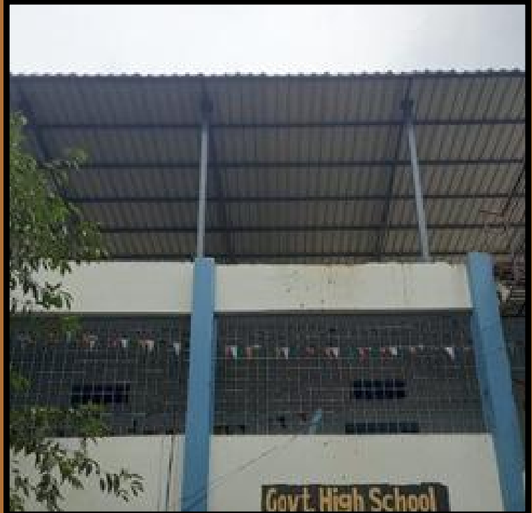
Rooftop work done in Shaikpet High School
